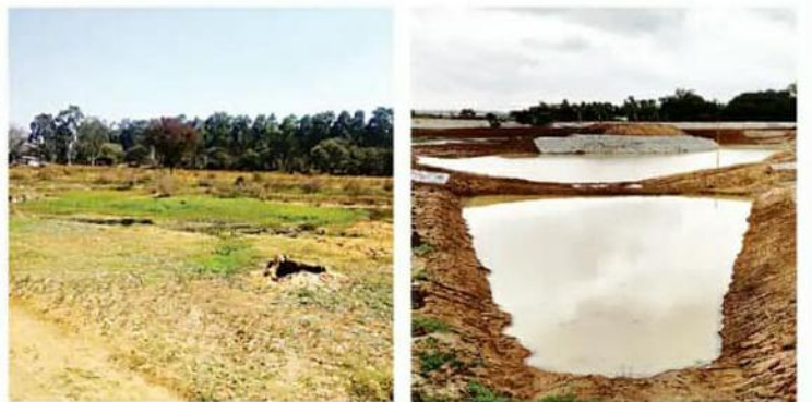
Before and after pictures of rejuvenation work at Vabasandra Lake at Bommasandra
